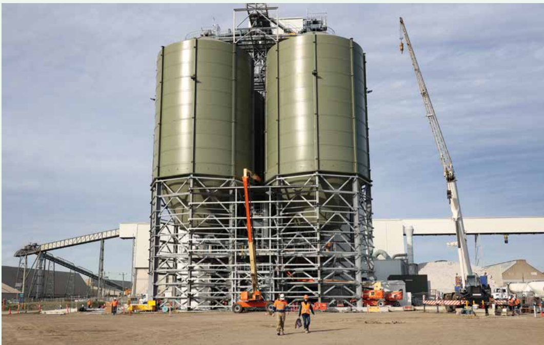
Geelong Cement grinding and storage facility, Vic
